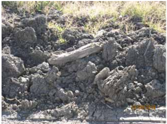
4. Issue: Unsuitable material in processing area on protected side of levee. GPS Coord: 2953.227 N 09008.606 W to 2953.249 N 09008.626 W
