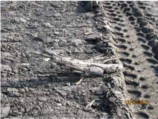
4. Issue: Unsuitable material in processing area on protected side of levee. GPS Coord: 2953.227 N 09008.606 W to 2953.249 N 09008.626 W
